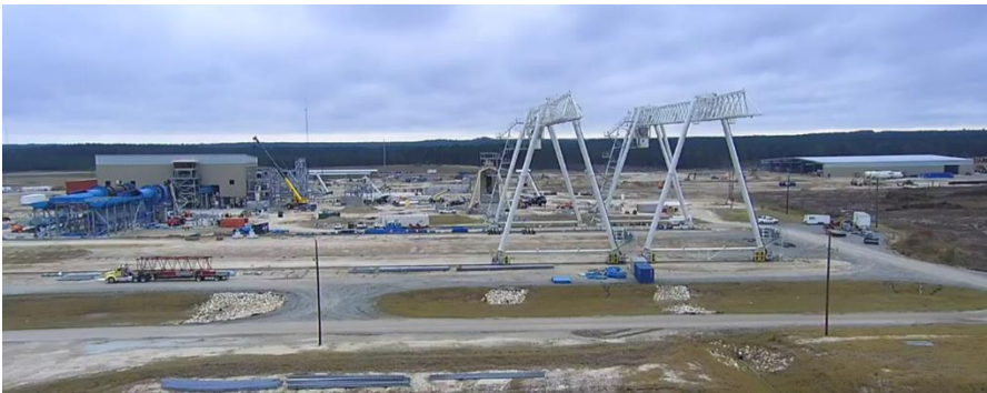
Aerial view of the Corrigan OSB, L.L.C. construction site, taken November 9, 2016
